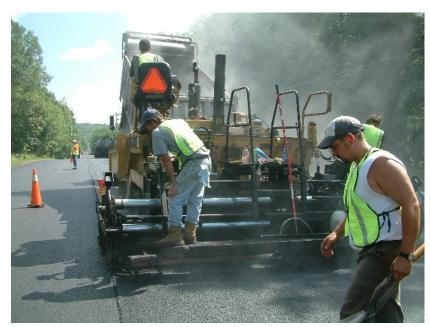
resistance, renews aging surfaces, fills micro-cracks, and seals and waterproofs the pavement.
