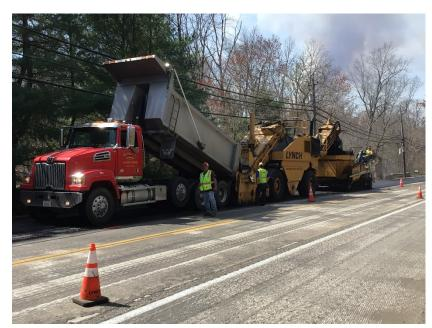
• Thin Overlay (Paver-Placed Elastomeric Surface Treatment - PPEST) — a one inch thick, gap graded hot mix with a modified asphalt cement. The modified asphalt greatly improves the mix's flexibility resulting in a more crack-resistant pavement.
