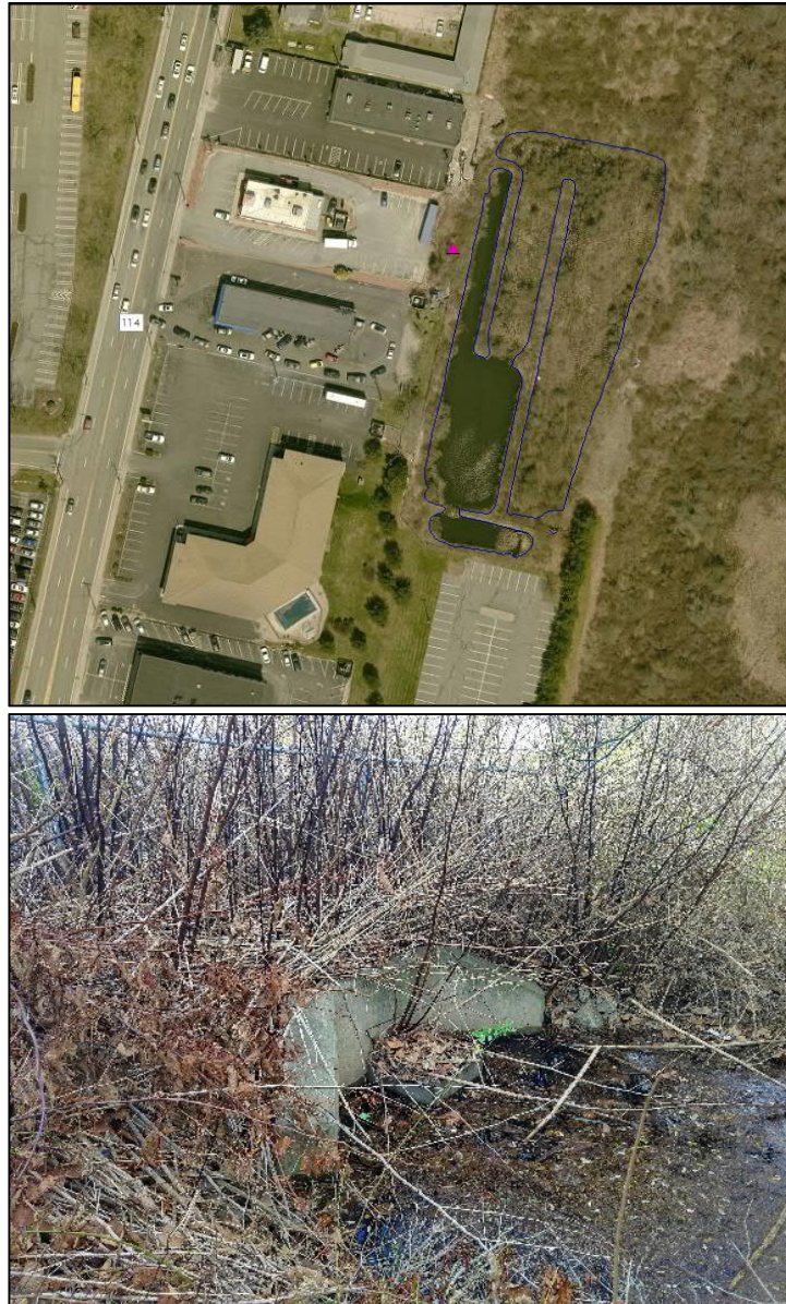
Photo 1: Top, aerial view of STU, pink triangle indicates RIDOT outfall mapped location. Bottom, outlet blocked by leaves and branches.
