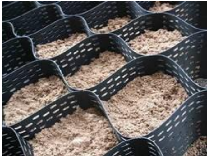
Figure 2. Typical Cellular Confinement System
