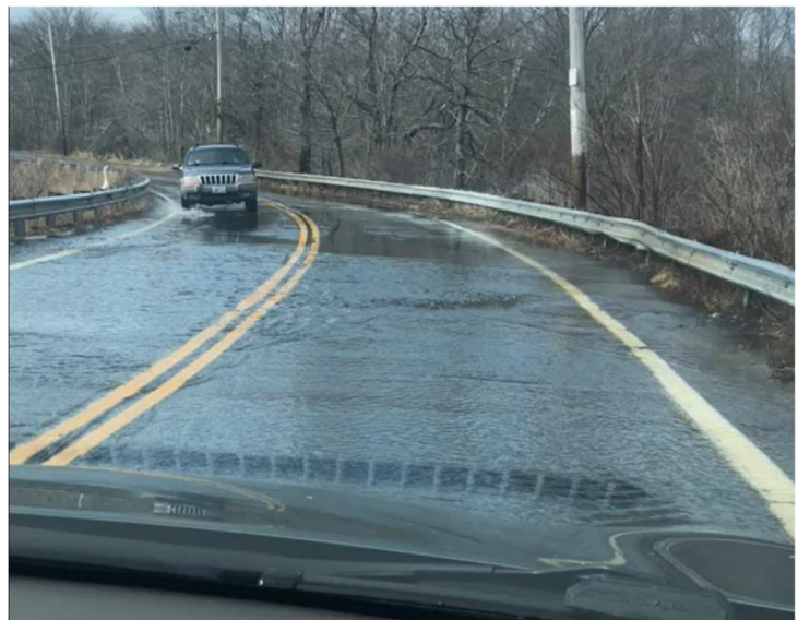
Figure 6: Schoolhouse Rd flooding during rain event (March 2018)
