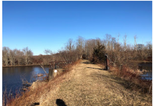
Figure 4: Upper Kickemuit River dam
