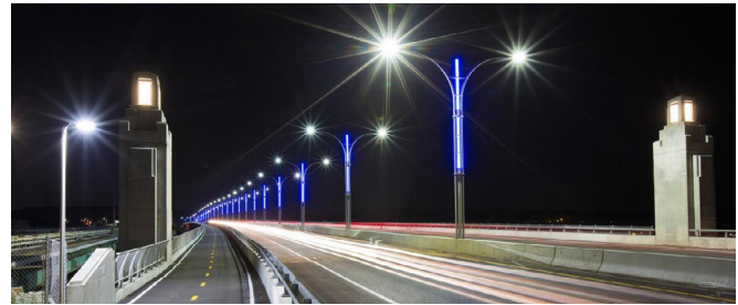
Sakonnet River Bridge
