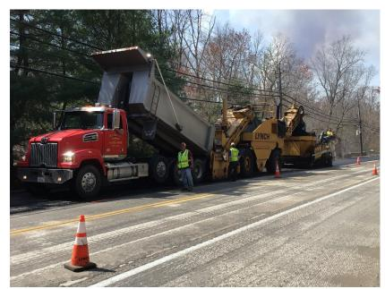
resistance, renews aging surfaces, fills micro-cracks, and seals and waterproofs the pavement.
