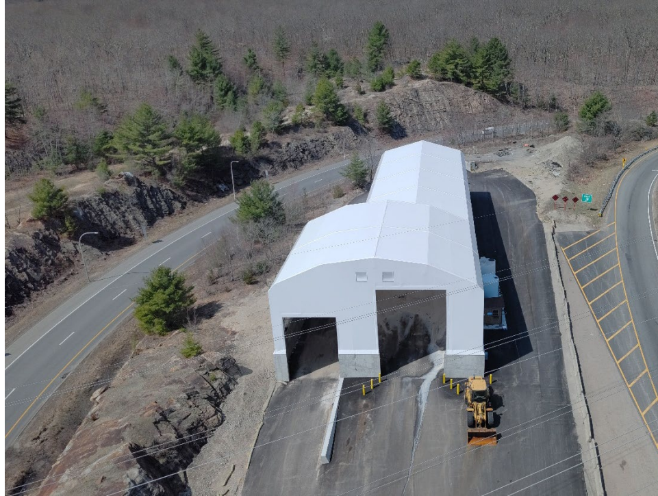
Salt Storage Facility - Johnston
