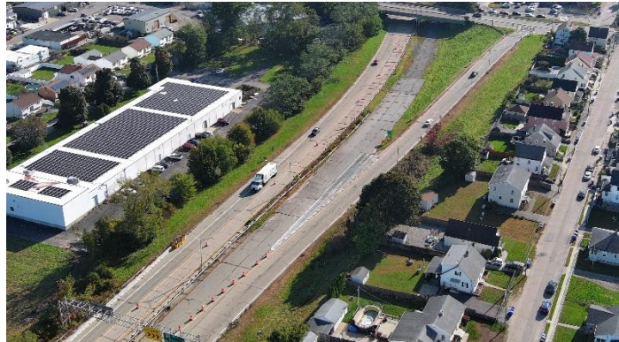
Figure 4-7 Aerial Photo, Henderson Expressway during Phase 1 Construction
