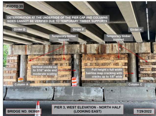
Figure 3-6 Inspection Photo, Bridge #638
