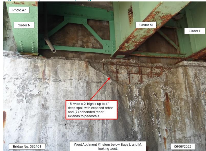
Figure 3-5 Inspection Photo, Bridge #624
