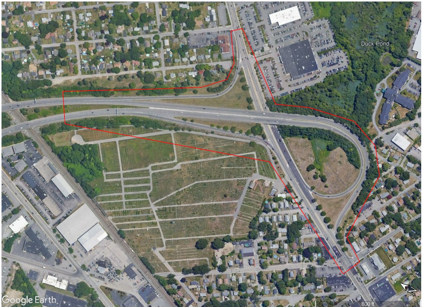
Figure 3: Existing Conditions at the Route 37 and Post Road interchange in Warwick, RI.
