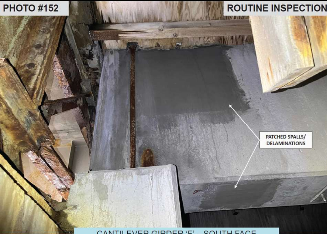
CANTILEVER GIRDER 'F' – SOUTH FACE AT PIER #7 IN SPAN #7 (LOOKING NORTH)
