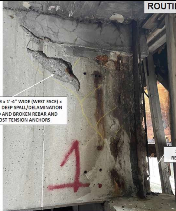
CANTILEVER GIRDER 'A' - NORTH FACE AT PIER #7 IN SPAN #7 (LOOKING SOUTH)
